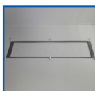
3 Knock Out Holes
